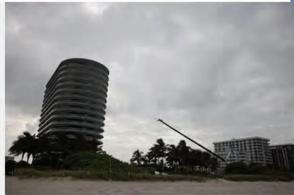
SITE OF THE CHAMPLAIN TOWERS SOUTH, WHICH COLLAPSED JUNE 24, 2021.
