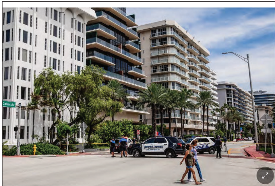
High-rise condominiums along Collins Avenue, near the site of the Champlain South Towers collapse in Surfside, Fla. Scott McIntyre for The New York Times
